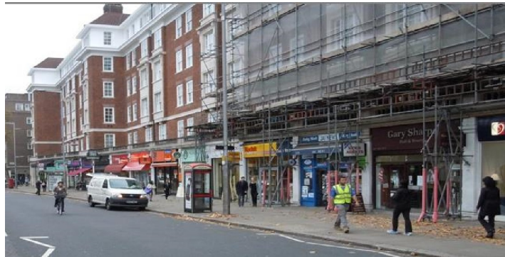
Photograph 1 - Existing Parking Restrictions (with Loading Restrictions) on Kensington High Street — close to Holland Green Place
