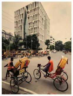
The Gulshan Society Mosque in Dhaka reimagines – and rearranges – mosque architecture with seven identical prayer halls stacked one on top of the other. The project's aim was to accommodate a large congregation on a small plot, while also providing an attractive landmark for the densely packed area. The building's outer pattern is an abstraction of a prayer in Kufic script.
